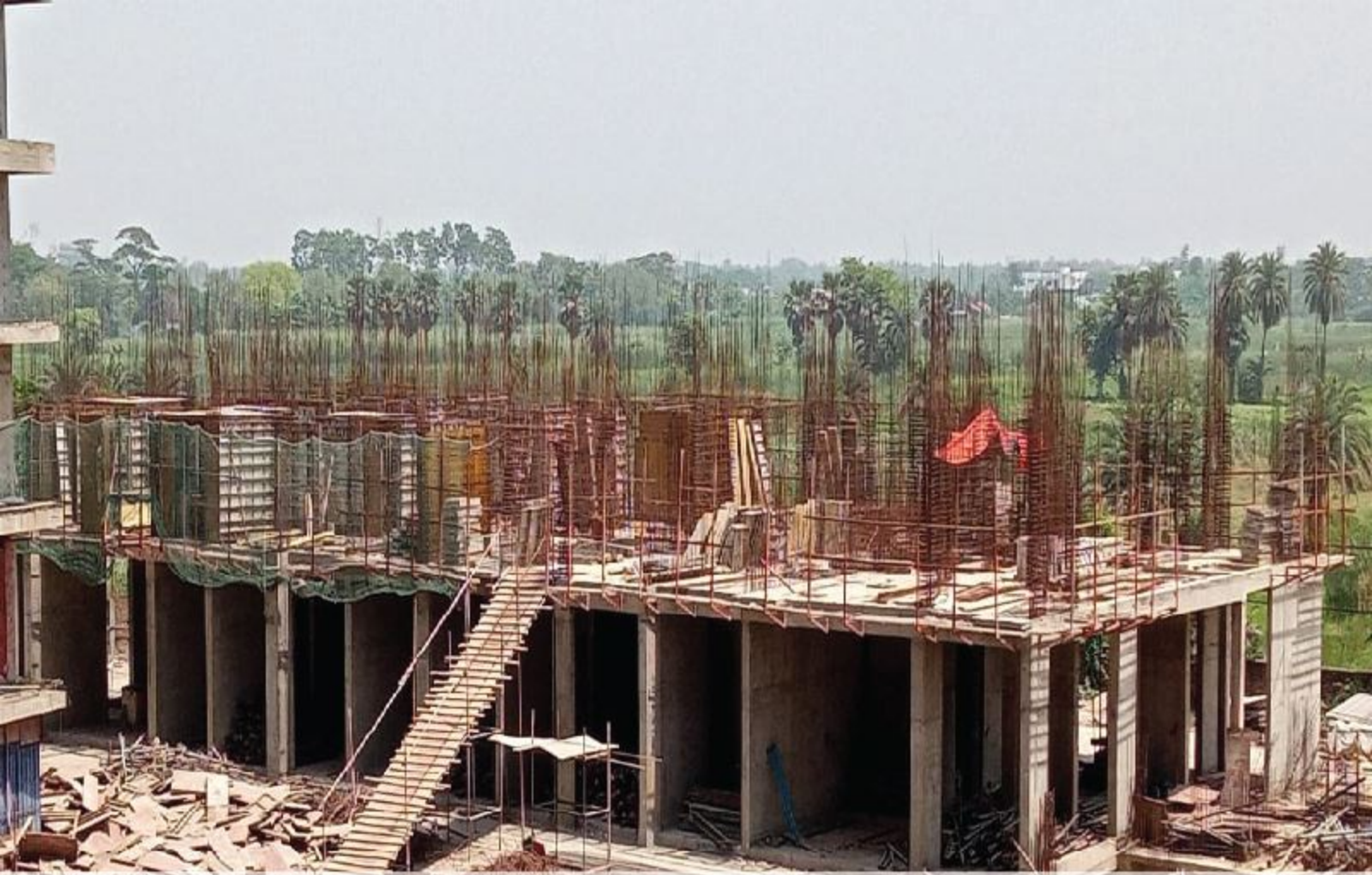
TOWER-10 (F):: Slab at 1st Floor Level Completed
